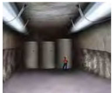
3: Resin Liner Shields within ILW emplacement room
