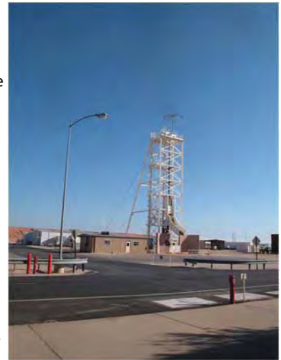
Headframe at Waste Isolation Plant, New Mexico
