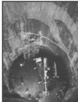
Excavating the caverns for the Lovisa facility in Finland
