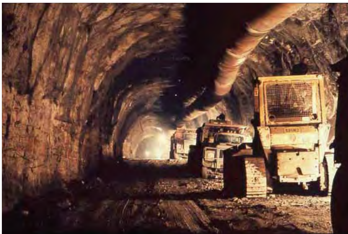
Construction during Darlington cooling water intake tunnel
