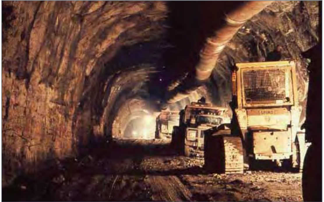
Darlington cooling water intake tunnel
