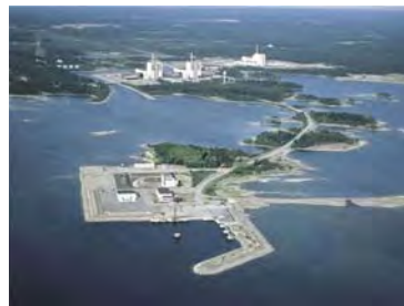
The SFR in Sweden manages L & ILW in bedrock caverns 60 metres below the Baltic Sea.
