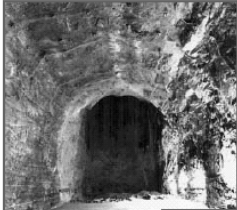
Cooling water tunnel at Darlington
