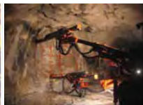
Excavation by drill and blast
