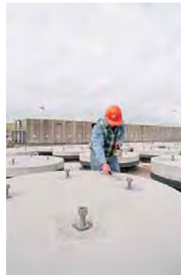
Intermediate Level Waste Storage
