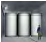
Resin liner shields within intermediate level waste room
