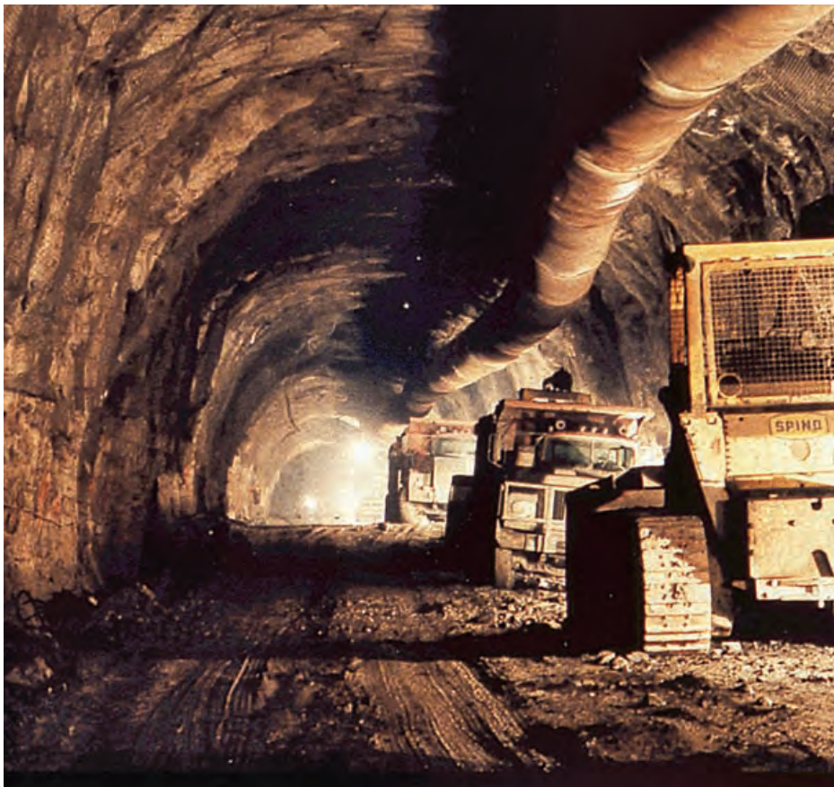
Construction of the cooling water intake tunnel at Darlington in the Cobourg Formation provided evidence that the formation can sustain a stable, dry opening
