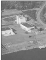
Surface facilities of Forsmark facility in Sweden
