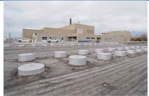
Intermediate level waste storage.
