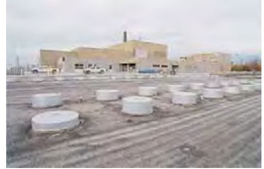
Intermediate level waste storage.
