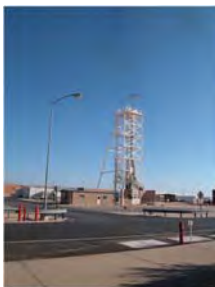
Headframe at Waste Isolation Plant, New Mexico
