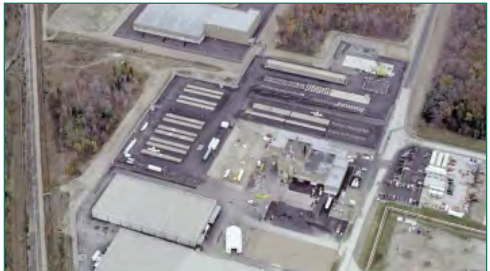
Aerial view of the Western Waste Management Facility at the Bruce site.
