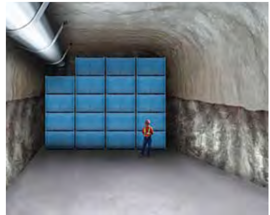
Low level waste emplacement room
