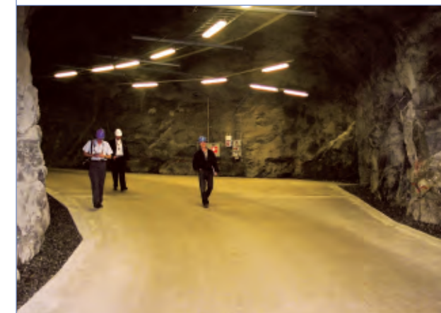
An emplacement room at the Waste Isolation Pilot Plant in New Mexico, United States, a facility which was constructed at about the same depth as OPG's DGR is planned.
